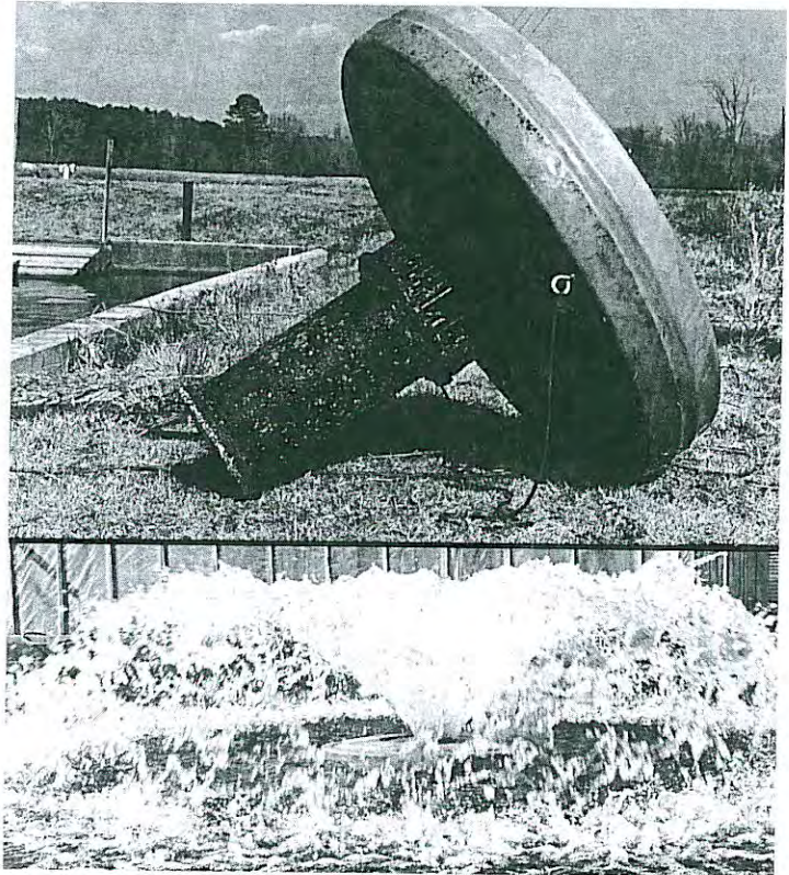
Figure 17. Vertical pump aerator.
